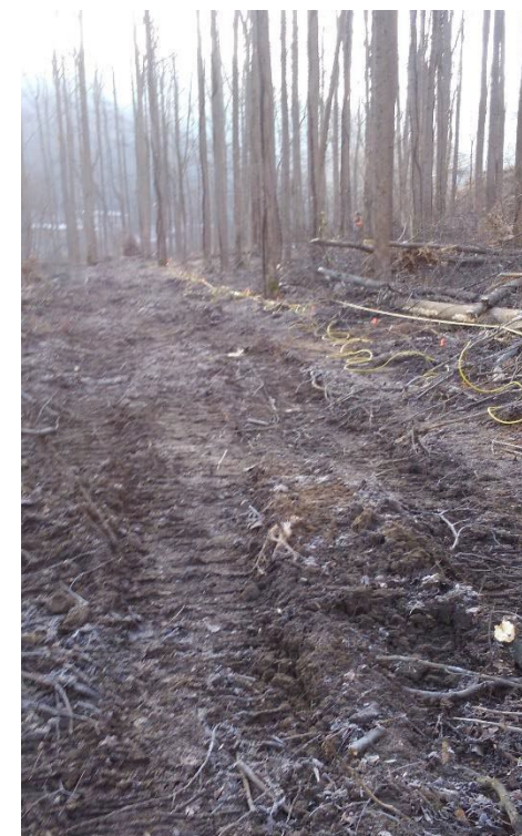
Figure 3. Image showing the site conditions as well as an ER line traversing from the top of the image to the right. Trees were felled to permit some access for geophysical surveys and heavy equipment operators for excavation.
